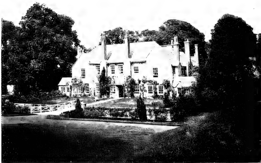
A SMALL HOUSE-COURT
